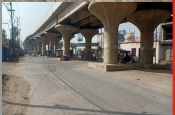
Railway Over bridge Rewa, MP
